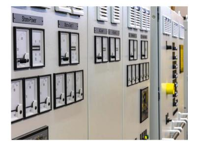
The link is set up in two distribution systems. In normal operation, these are interconnected. If a fault occurs in one part of the link supply, it is disconnected. The non-defective part of the link supply can continue to be operated. The links are monitored by two insulation monitors. Link is set up to be selective according to the DNV and the Estrin 2025 regulations.
